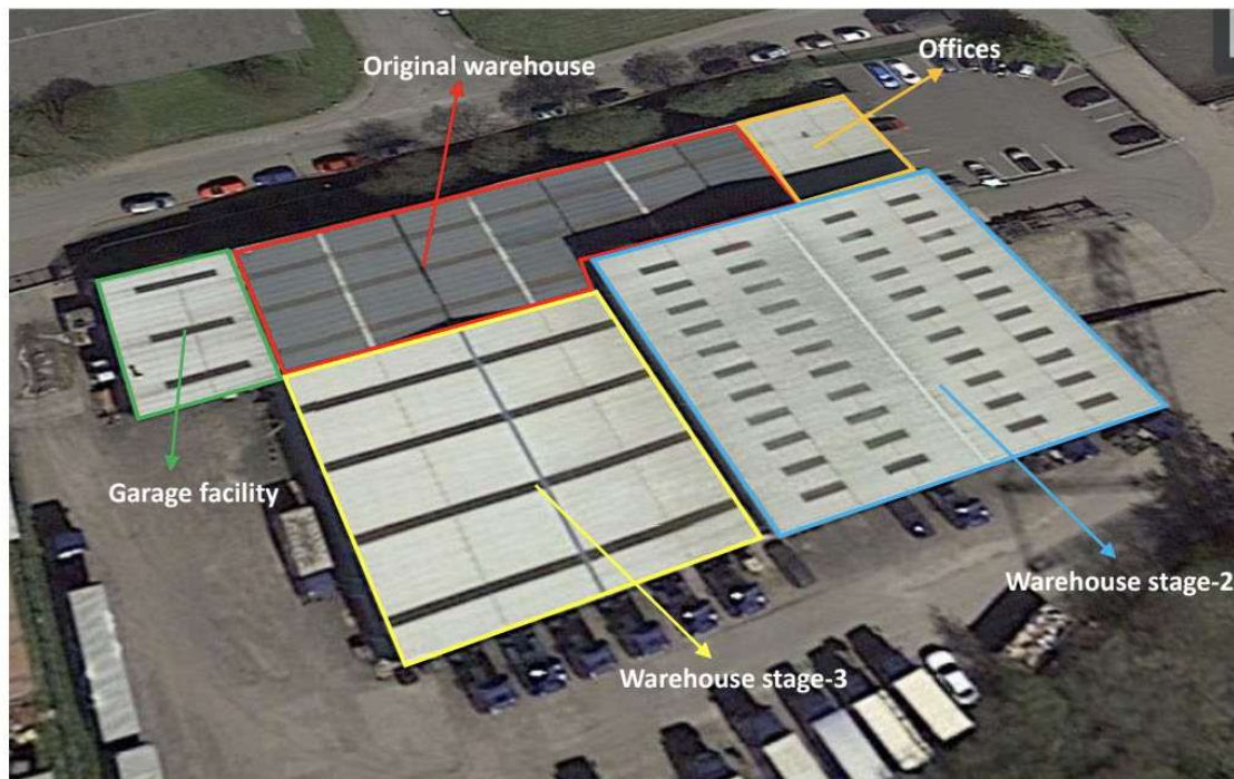
Figure 1. Google map view of the buildings at KB Event site in Pinxton
